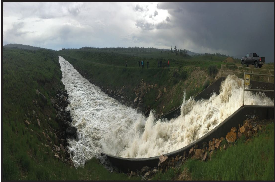
Azotea, San Juan-Chama Project
