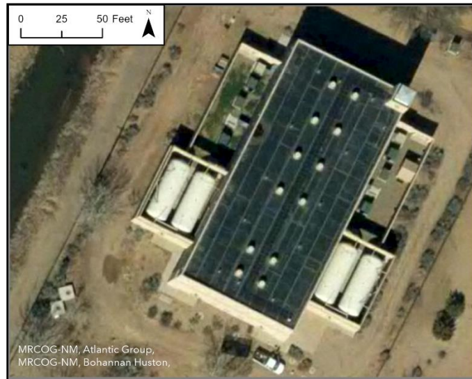
Figure 5-4: Raw Water Pump Station Aerial View
